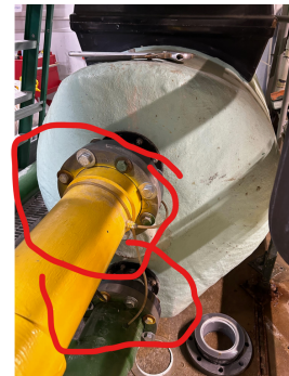
Sand filter flange after being capped off
