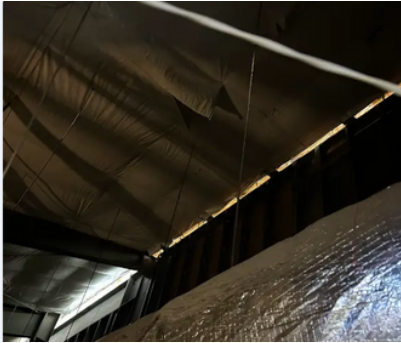
Wall between the pool & cardio room
